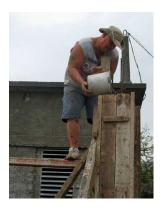
We mix the concrete with one bucket of cement, three of sand and two of gravel. We then bucket by bucket fill the columns.
