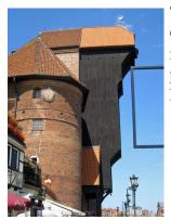
The Great Crane is the most characteristic and unmistakable symbol of Gdansk. In the Middle Ages it was the largest port crane in Europe. The reconstructed mechanism inside is still in working condition and is powered by men in an immense wooden wheel who would walk in it like hamsters.
